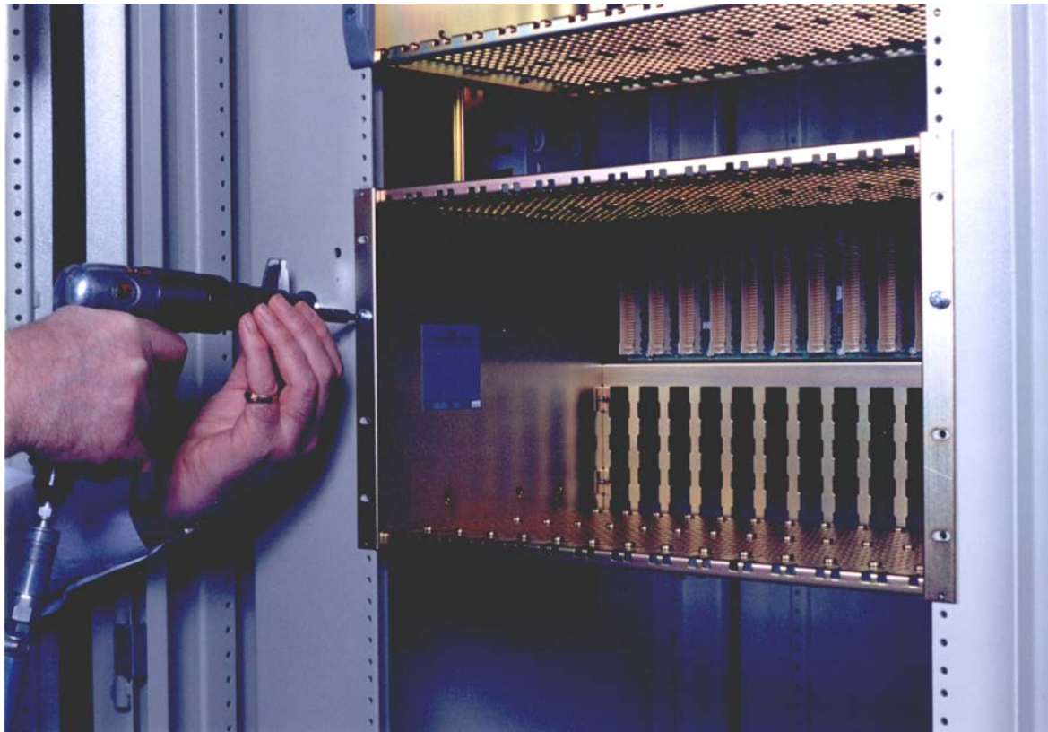
Figure 9 Installation of Chassis
